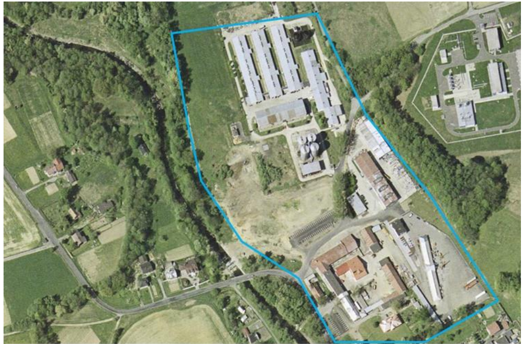
Figure 6. The case study area in an aerial photograph at the start of the regeneration process (e.g., prepared new parking lots) in 2003. The boundary is marked by the blue line. Source: [61].
