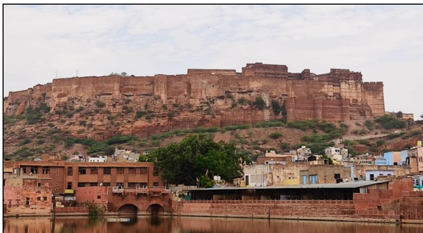
Figure 5. The Mehrangarh Fort built in Jodhpur Sandstone located over the Jodhpur group of Malani-Igneous Suite (Source: Authors' own)
