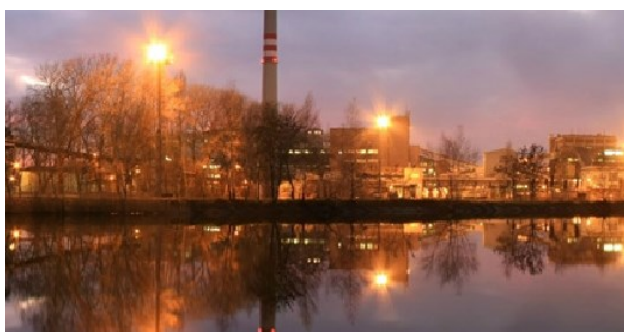
Fig. 1. Coal heating plant in the Czech Rep. [15]
