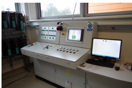
Fig. 1. Controlling board for duct tract
